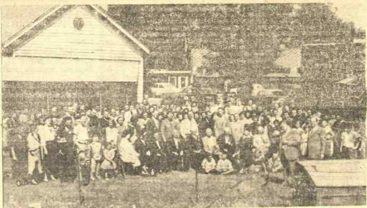
Shown above is a portion of the Sunday morning congregation of Iuka Baptist Church, which attended the Ground Breaking services held October 5th for the new Educational Building. Seated in chairs are the oldest members. Sitting on the ground are the youngest members. Ages range from 6 to 98 years. The group of men standing back of the chairs compose the building committee, of which Mr. W. C. Hundley, holding the shovel, is chairman. Plans have been adopted and construction will start soon.
